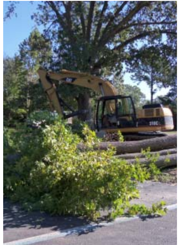
Construction on the addition to the Suffolk Children's Center began in October of 2011 with demolition.
